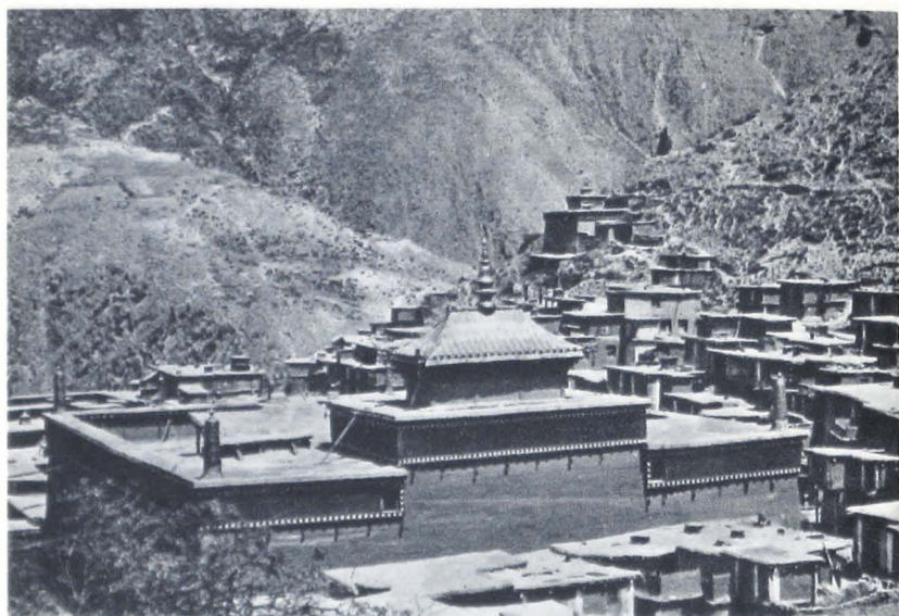
(a) The building which houses the printing-press at Derge
